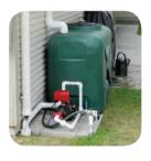
The **City of Abbotsford** uses a 35,000 litre storage system to harvest up to 868,000 litres of rainwater per year. This water is used for Parks and Works irrigation.
